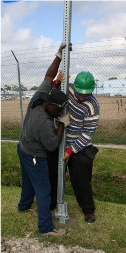
8. Lift and insert the post into the casting. Align the sign facing traffic. Insert a 3/8" X 3 1/2" shoulder bolt through one slot of holes in the casting and post. Attach a flanged hex nut and tighten. Repeat with other set of holes.
