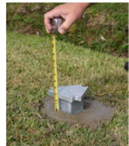
Level the base to make sure it does not drift off level while concrete sets.
