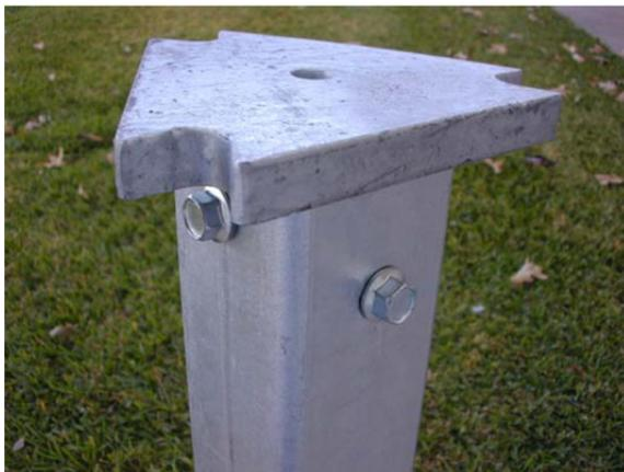
5. Center the anchor in the hole and slowly press it down until the stub triangular plate is a maximum of 3" from the ground line. Properly align the anchor to oncoming traffic. This will ensure that when the casting and post are attached the sign will be correctly aligned to traffic.
