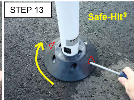
Place the threaded stub on the receptacle and tighten snugly with a Phillips screwdriver or similar tool.
