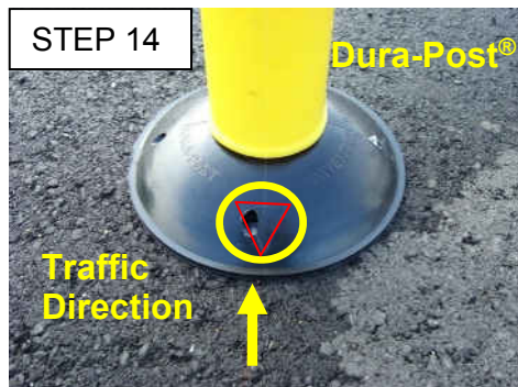
Place the threaded stub on the receptacle and tighten snugly with a Phillips screwdriver or similar tool.
