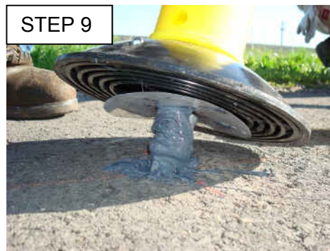
STEP 9 Place the post/anchor assembly into the hole.
