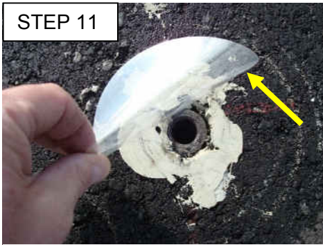
Unscrew the post and remove the adhesive shield and discard.
