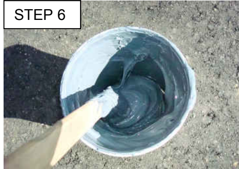
STEP 6 Thoroughly mix the epoxy.
