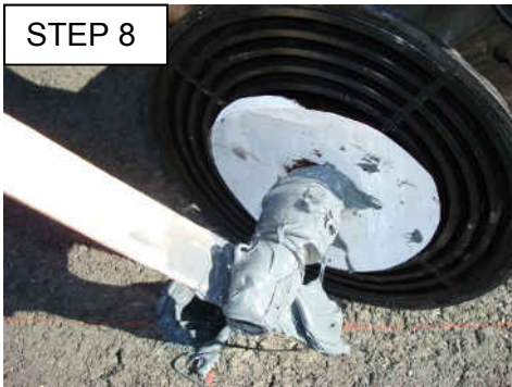
STEP 8 Coat the anchor with epoxy.
