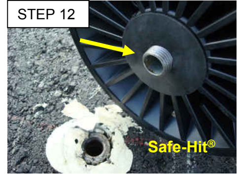
Place the 2-1/2" neoprene washer over the screw on the base. The washer prevents the base from rotating during service.
