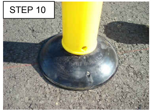
STEP 10 IMPORTANT!! Let the post sit until the epoxy fully cures (approximately 8 hrs).
