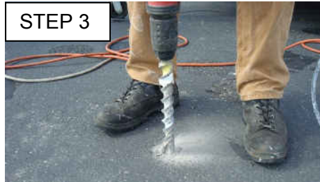
STEP 3 Drill 1-1/2" Diameter x 3-1/2" Deep. Consult OSHA respiratory standards for crystalline silica exposure.
