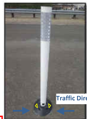
Completed SAFE-HIT® Post
