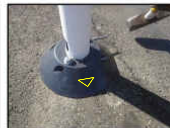
Place post in base and drive pins into place to secure post.
