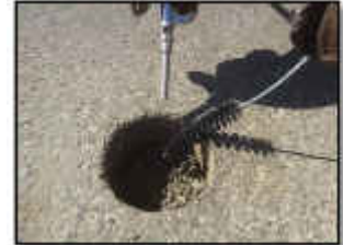
Brush and blow debris from hole.
