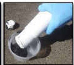
Use mixing stick to push epoxy into container. Thoroughly mix both parts to a solid gray consistency with no black or white streaks.
