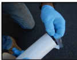
Remove cap from one end of both epoxy tubes.
