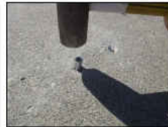
Place Anchors in holes and tap in with hammer.
