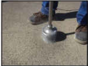
Drill 4" hole X 1 7/8" deep for SST Drill 4" hole X 2" deep for SLT
