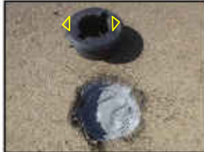
Pry out core section.
