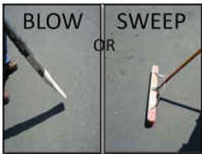
Sweep or blow area of debris
