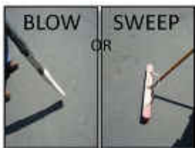
Clean area of debris with blower or broom.
