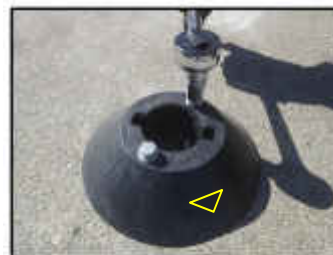
Secure base to concrete or asphalt with socket wrench and bolts.
