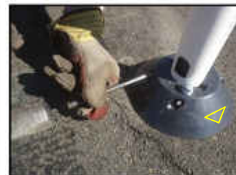
Complete driving the pins using a pin punch.
