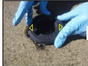
Chisel out remaining material from hole.
