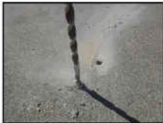
Drill 5/8" X 2 1/2" deep for Lag Shield Anchors (asphalt) or 1/2" X 1 5/8" deep for Drop-ins.
