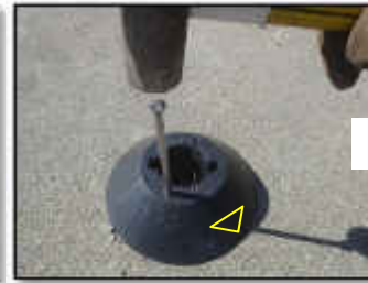
Use spike or 1/4" carbide drill to mark hole locations with arrows oriented in direction of traffic.
