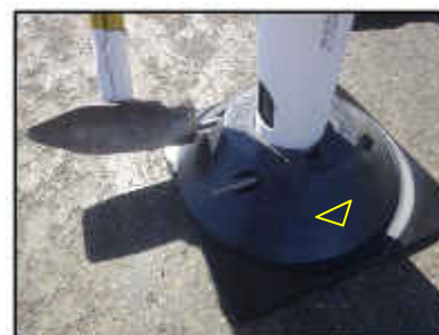
Place post in base and drive pins into place to secure post.
