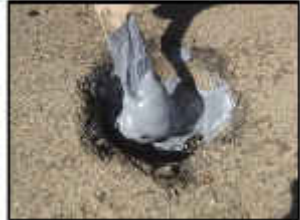
Drill 4" hole X 1 7/8" deep for SST Drill 4" hole X 2" deep for SLT
