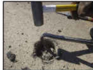
Chisel out remaining material from hole.
