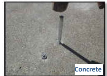
Set Drop-in Anchors with anchor setting tool.
