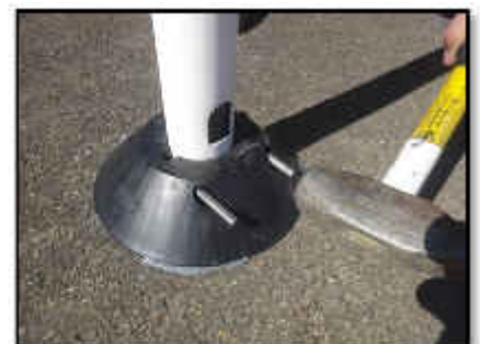
Allow the epoxy to set up, then place the post into the base and tap pins till flush with base (see note).
