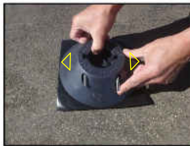
Place newly exposed side with arrows oriented with the direction of traffic.
