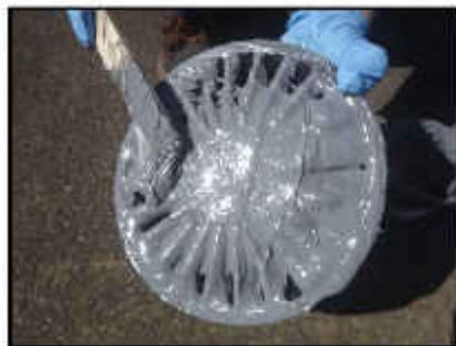
Apply epoxy evenly to bottom of base with stir stick.
