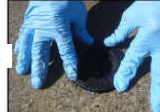
Brush and blow debris from hole.
