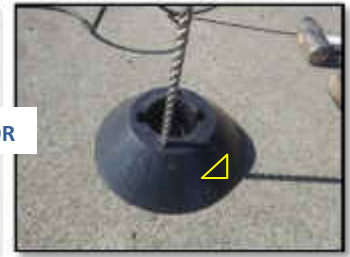
Use spike or 1/4" carbide drill to mark hole locations with arrows oriented in direction of traffic.
