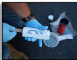
Use mixing stick to push epoxy into container. Thoroughly mix both parts to a solid gray consistency with no black or white streaks.
