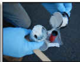
Remove cap from one end of both epoxy tubes.
