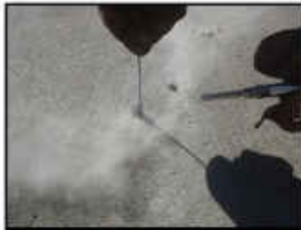
Use appropriate brush and compressed air to clear hole.
